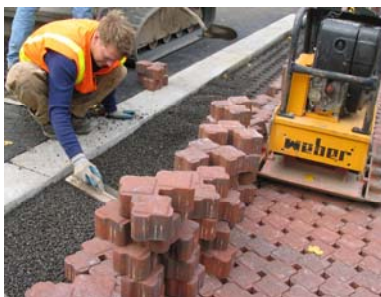
Ungrouted modular pavers are an example of a hydrologic source control (Source: Portland, OR).
